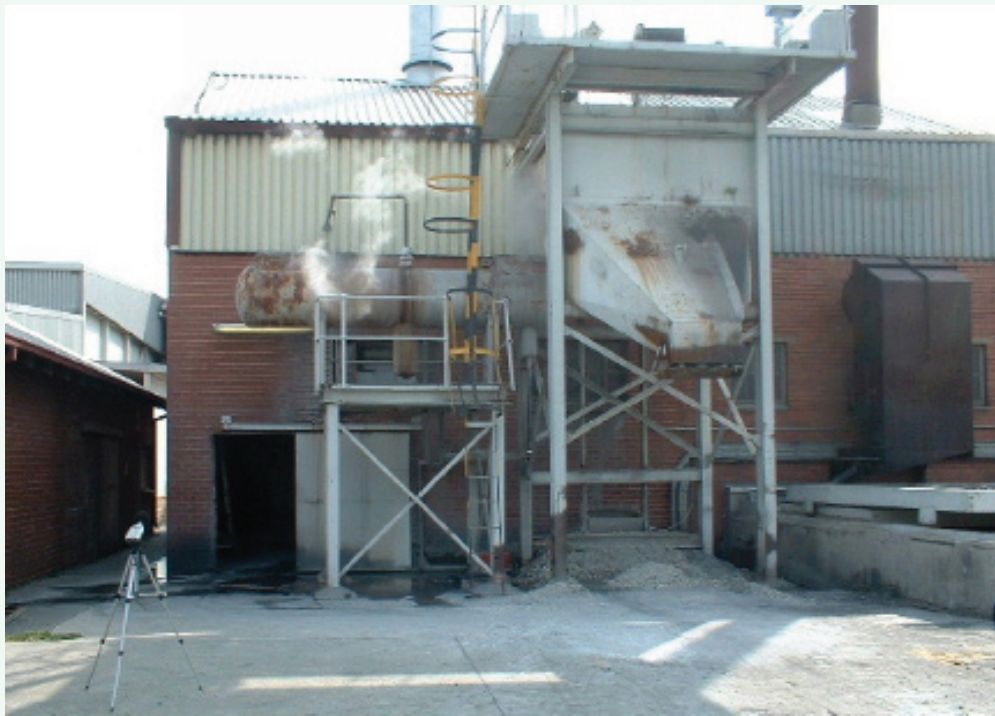
Abattoir 3 -View of boiler house
