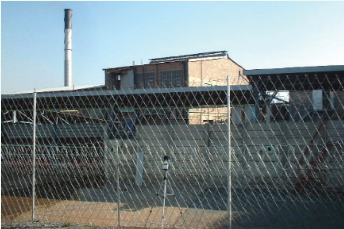
Abattoir 1 – View of boiler house across lead-in passage from stockyard to plant
