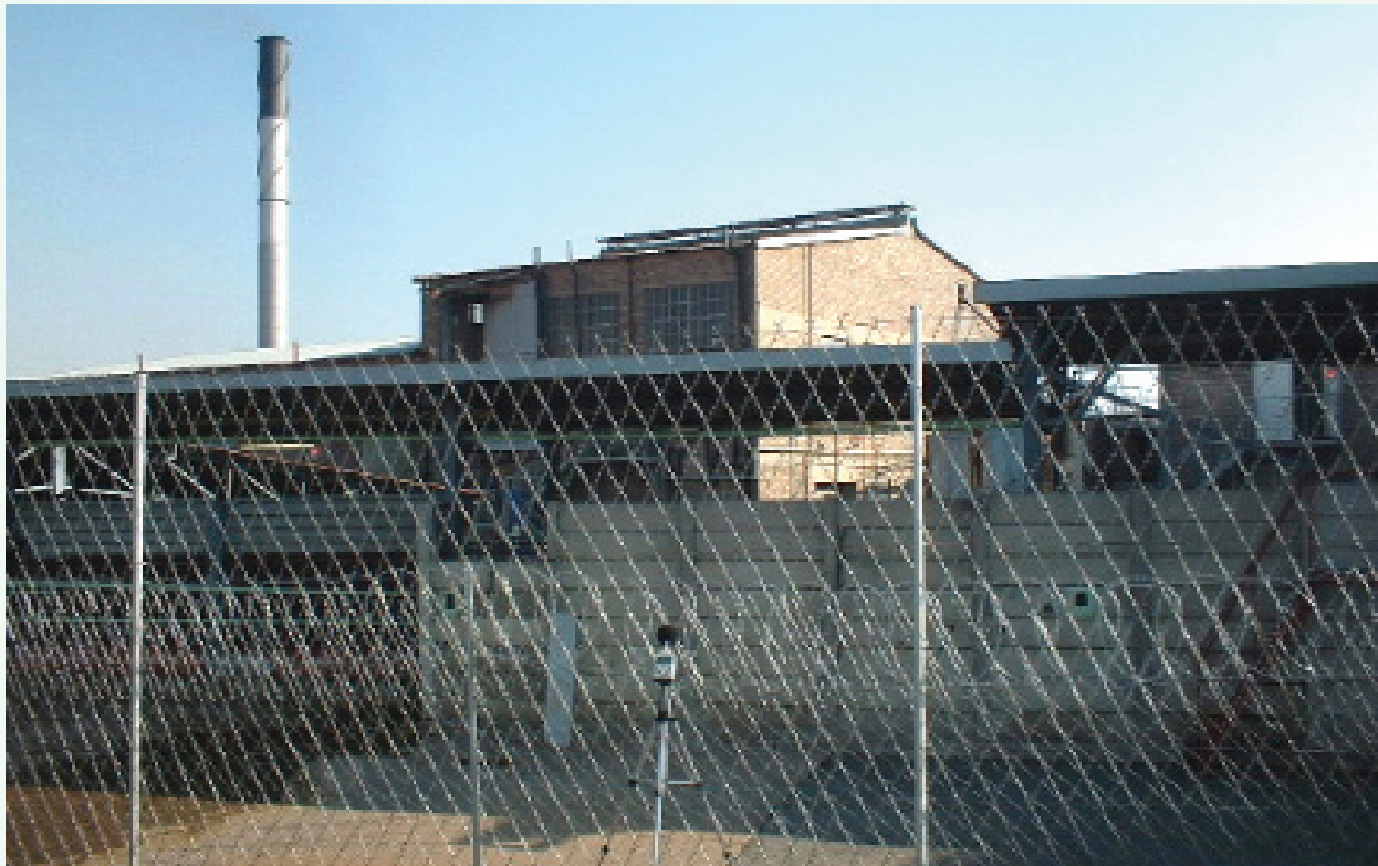
Abattoir 2 – View of ventilation fans and measurement position
