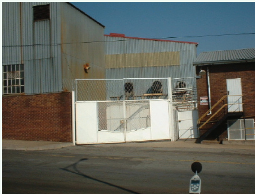
Abattoir 1 – View of ventilation fans from measurement position
